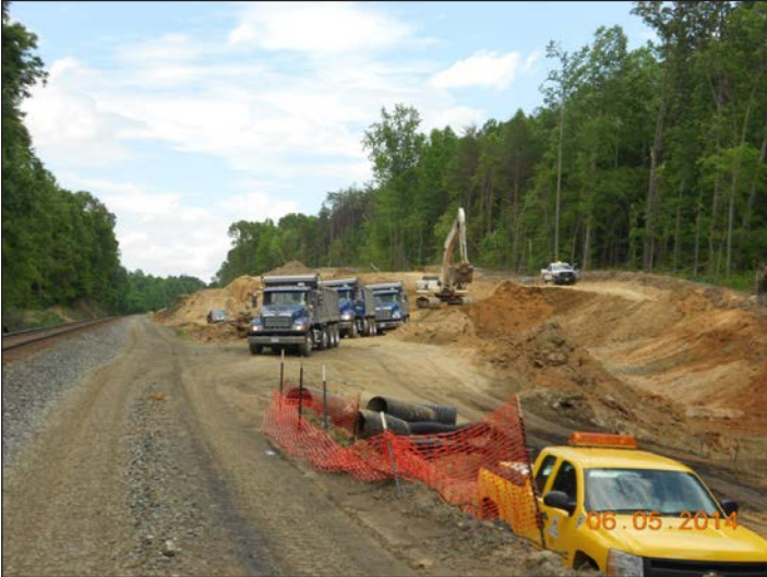
C-4901 Bowers to Lake - roadbed work
