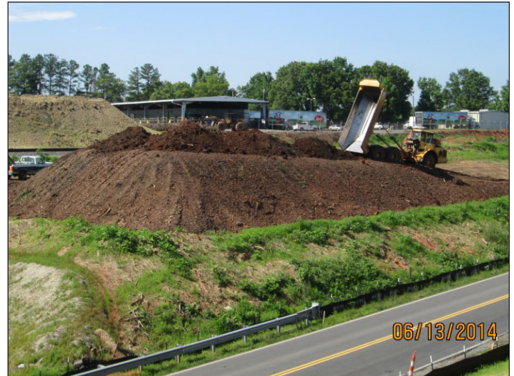
P-5208 Haydock to Junker - Grier Road Road Overpass
