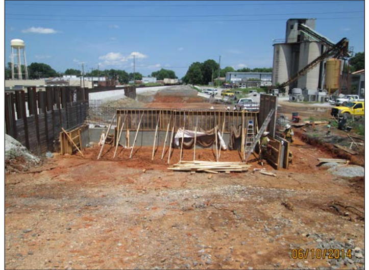
U-3459 Klumac Road - concrete form
