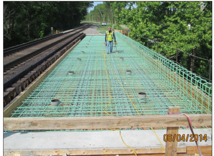
P-5208 Haydock to Junker - Rocky River Bridge
