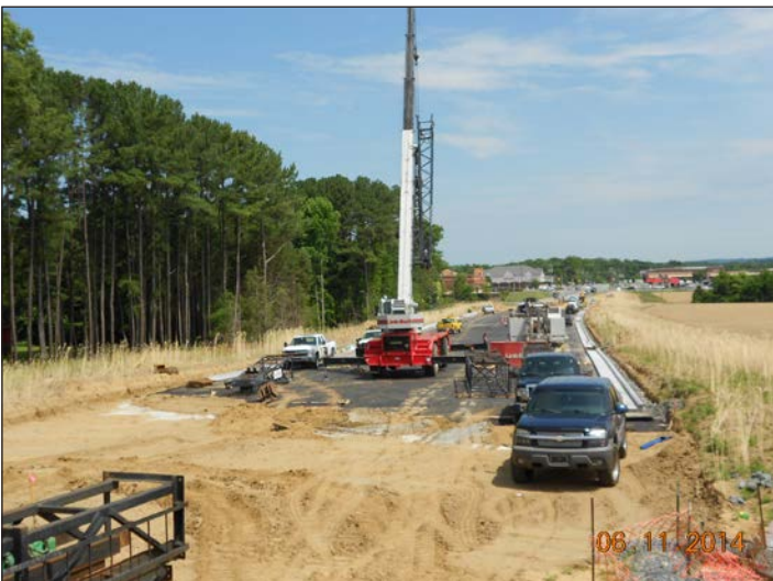
P-5208 Haydock to Junker - Roberta Road overpass
